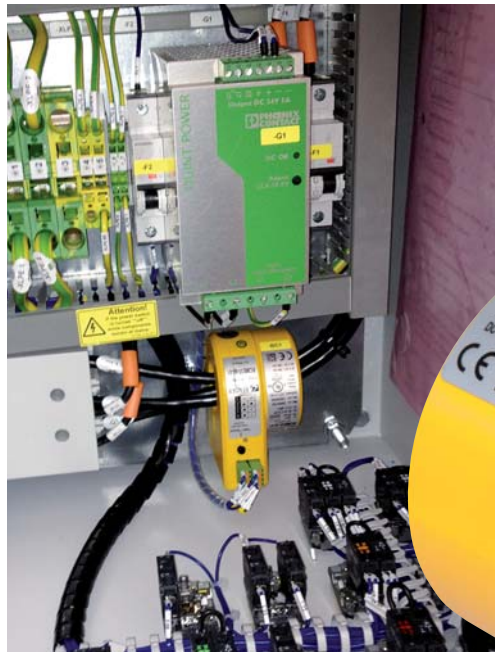
RCMB35-30 to enhance the electrical safety in welding systems
